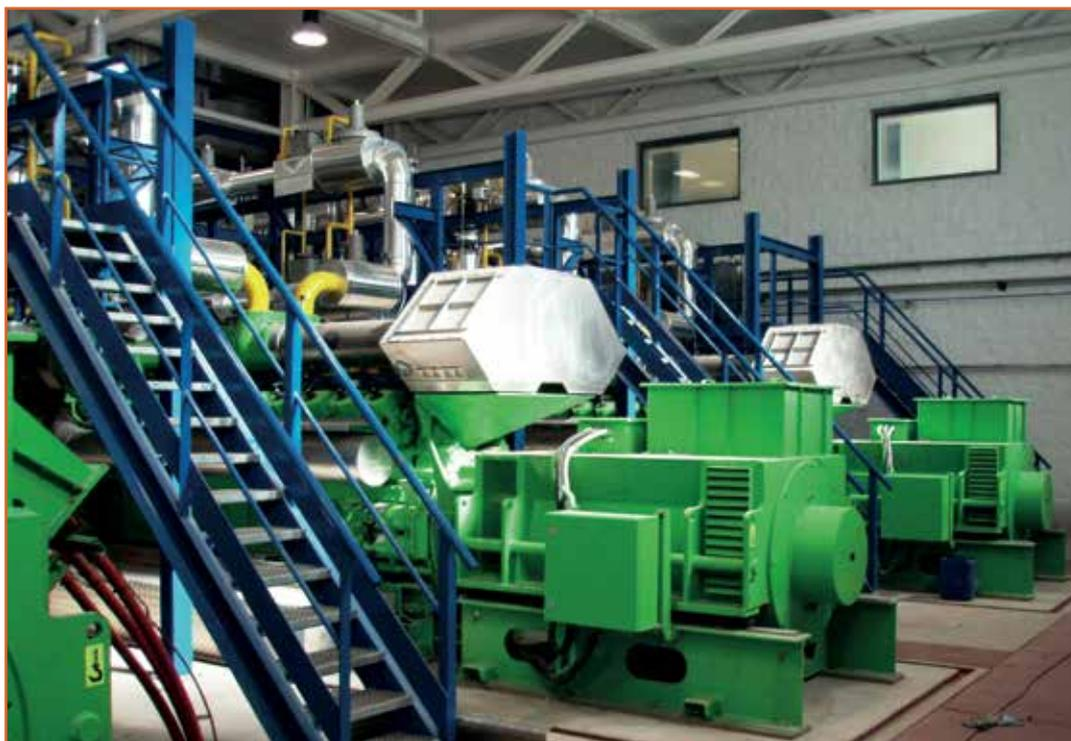
6 MWe syngas engine generator room at Eqtec's Movialsa plant in Spain
